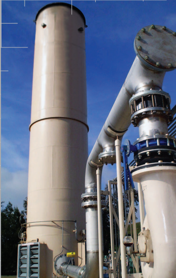
Photo courtesy of LFG Specialties
